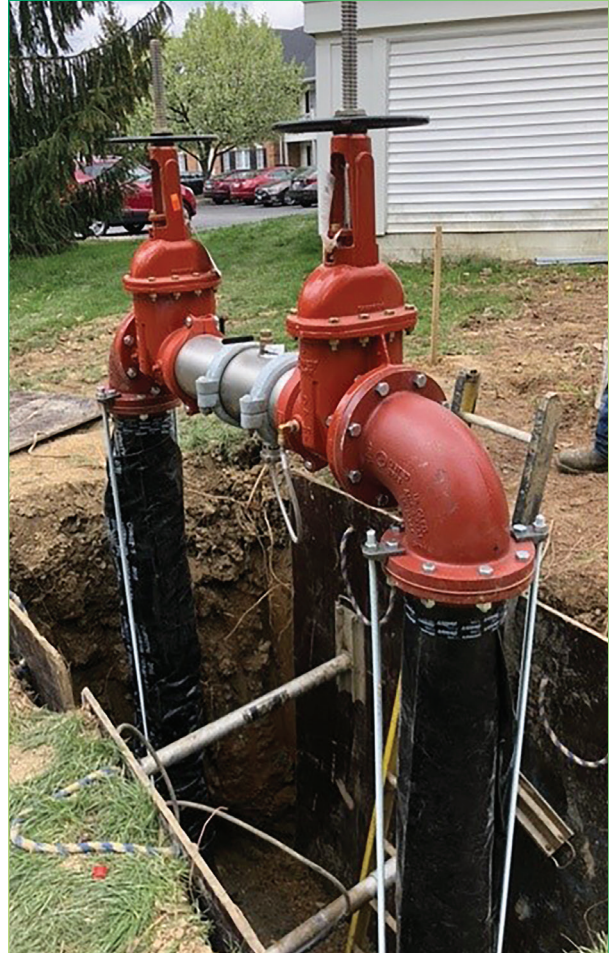
Preliminary installation of Double Check Valve at a Condominium Complex
